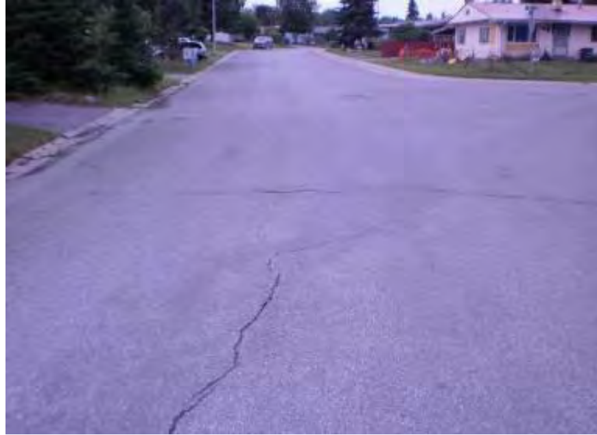
Figure 4-5. 19th St, Anchorage, chip seal applied in 2001, photo taken in 2011
