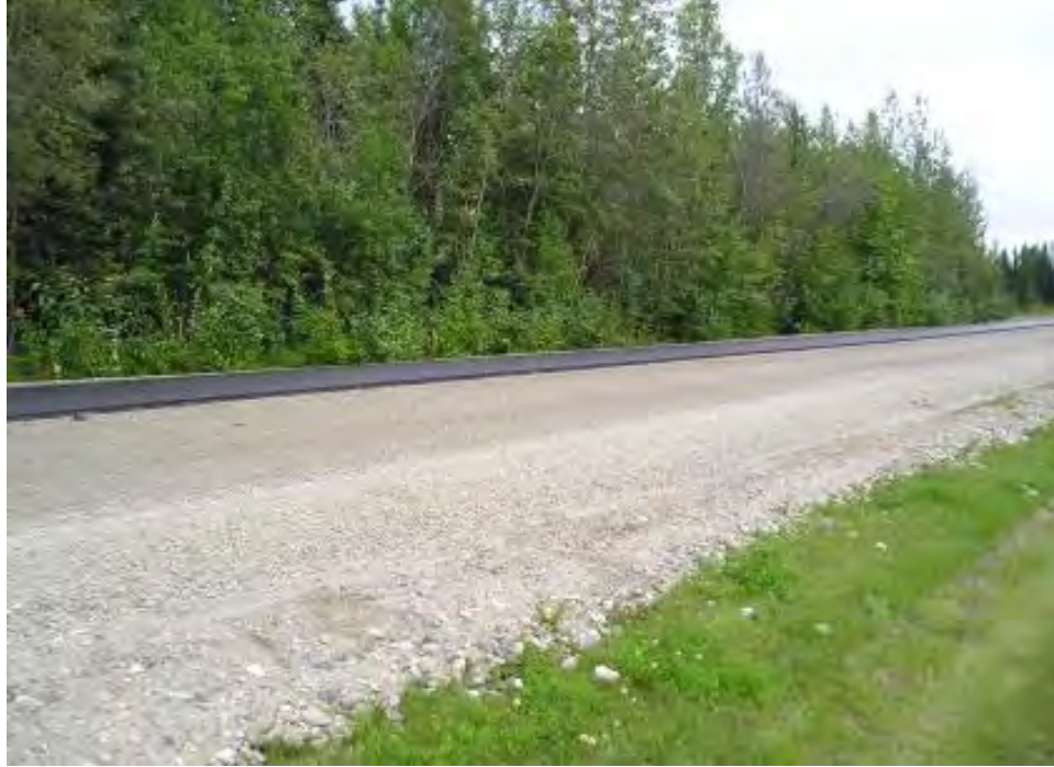
Figure 4-15. H & H Blvd, North Pole during thin HMA overlay construction
