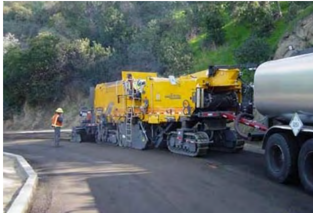
Fig. E.4 Cold-In-Place Recycling Machine
