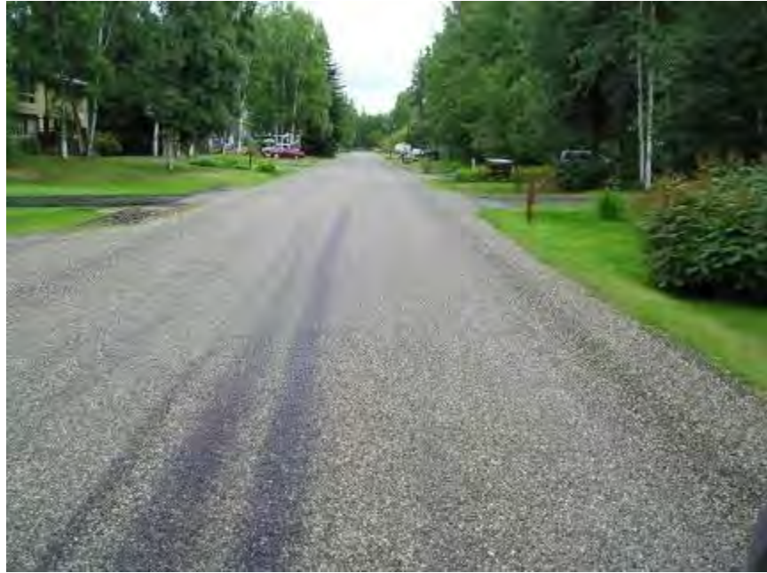
Figure 4-37. Teal Ave between Fairbanks St and Ramola St, Fairbanks, single C chip AST applied in 2011, post application, photo taken in 2011
