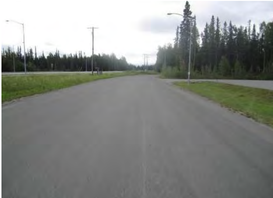
Figure 4-19. Slurry seal, Chief Thomas Dr., Fairbanks, applied in 2003, photo taken in 2011
