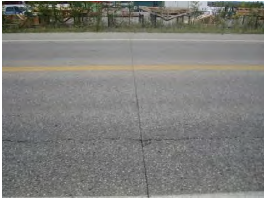
Figure 4-59. Philips Rd, Fairbanks, pre-saw cut joints applied in 2000, no sealing, photo taken in 2011
