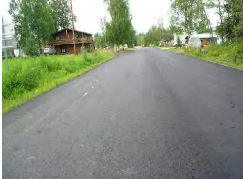
Figure 4-13. Davis Blvd, North Pole just after thin HMA overlay placed 2011
