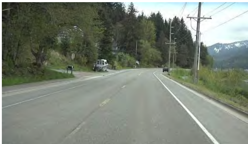
Figure 4-4. Twin Lakes Rd, Juneau, Chip seal placed in 2006. Photo from the Dynatest vehicle in 2010
