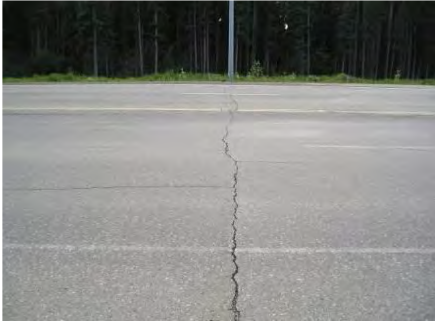
Figure 4-15. Farmers Loop Rd between Ballaine and Tanana, Fairbanks, double chip seal applied in 2008, thermal cracking and degrading permafrost, photo taken in 2011
