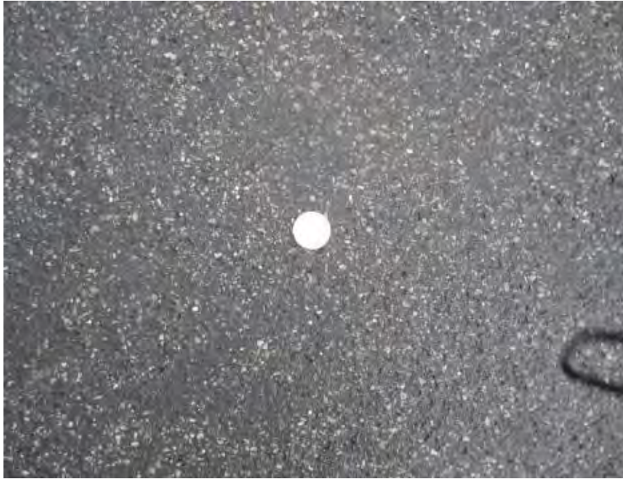
Figure 4-3. Eielson Air Force Base microsurfacing application, photo taken in 2011
