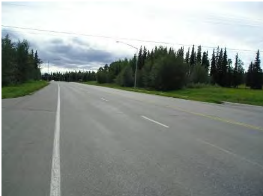
Figure 4-14. Farmers Loop Rd between Scenic Hts and Ballaine, Fairbanks, double chip seal applied in 2008, thermal cracking, photo taken in 2011
