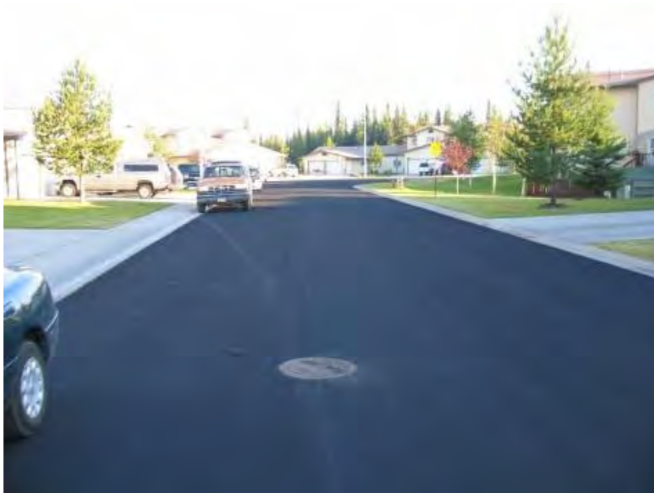
Figure 4-2. Eielson Air Force Base after microsurfacing application in 2003
