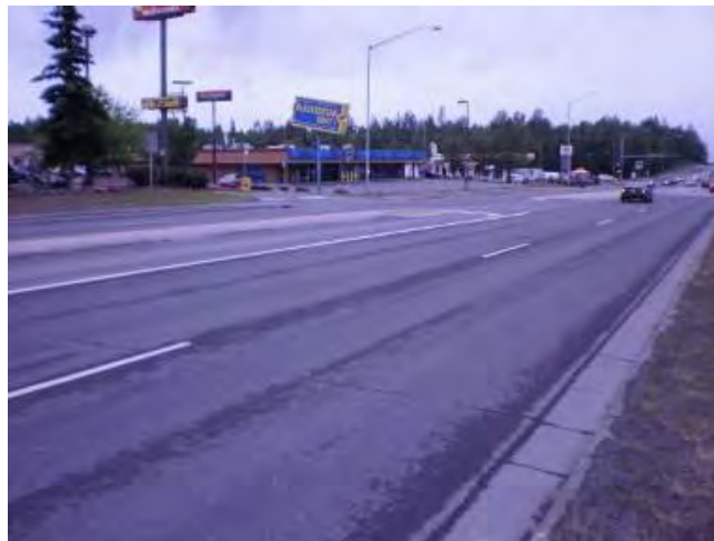
Figure 4-2. Debarr Rd, Anchorage, thin HMA overlay, placed in 2010
