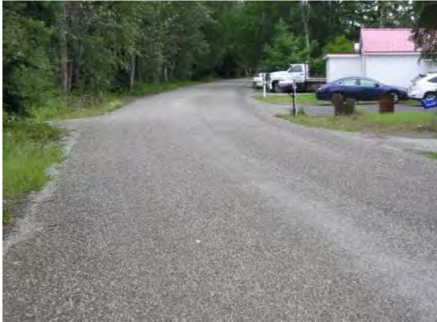
Figure 4-20. Mack Blvd between Morgan Way and Old Pioneer Way, Fairbanks, single C chip AST (post application), 2011
