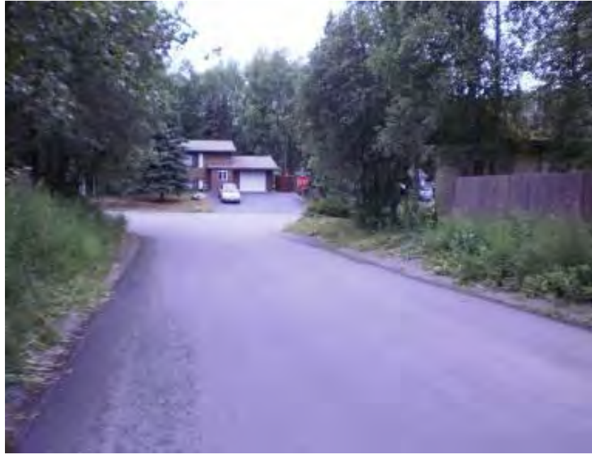
Figure 4-7. Duben St, Anchorage, chip seal applied in 2001, photo taken in 2011
