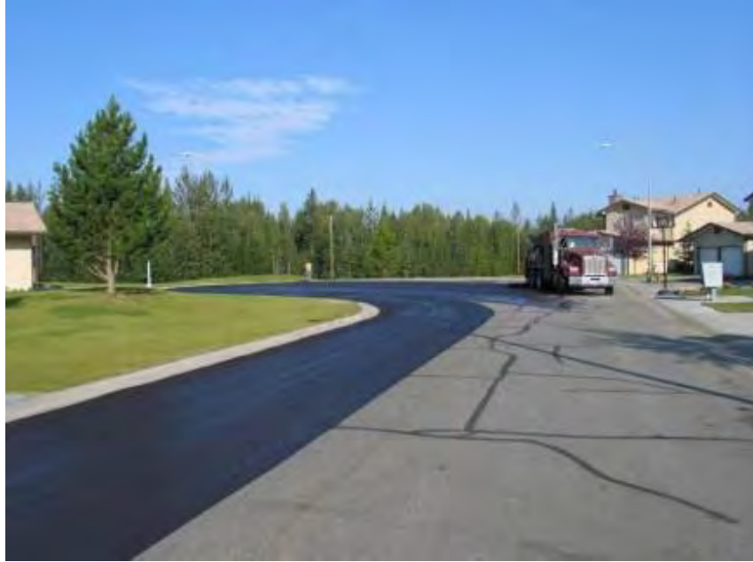
Figure 4-1. Microsurfacing being applied at Eielson Air Force Base in 2003
