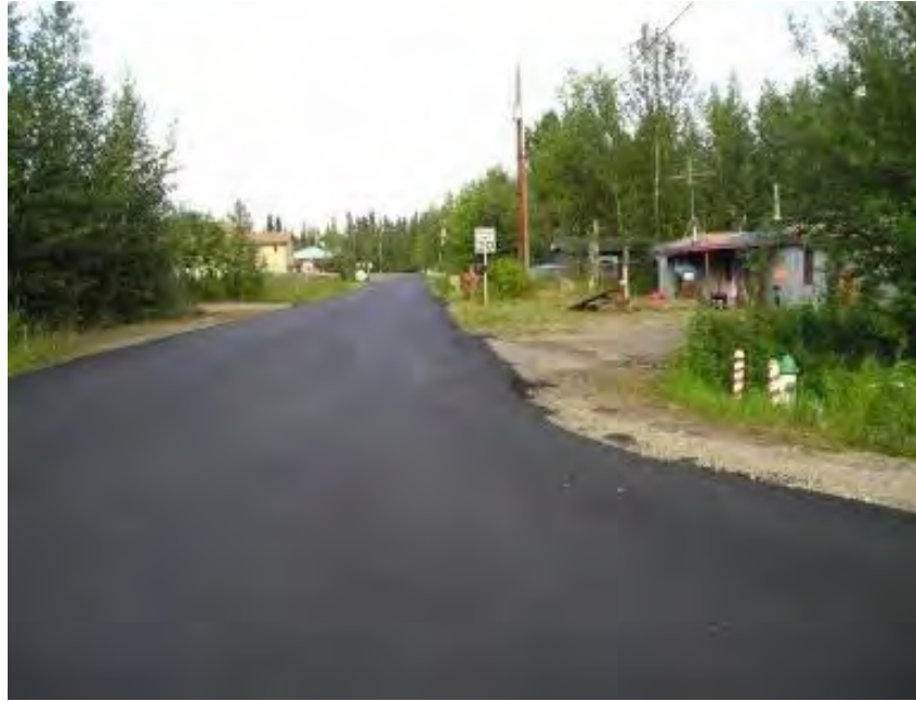
Figure 4-7. Cross Way, North Pole, just after thin HMA overlay, 2011
