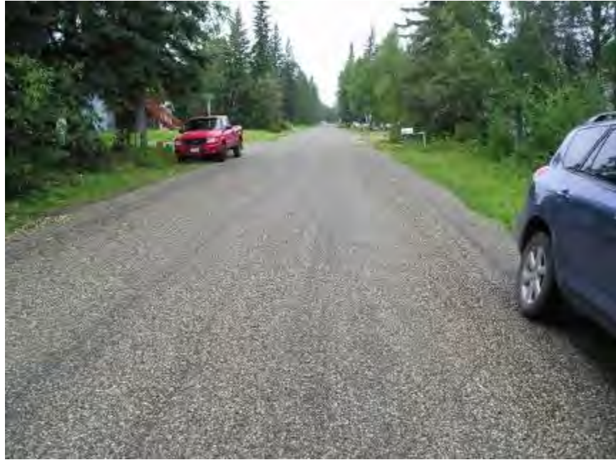
Figure 4-43. Old Pioneer Way between Luke St and Mack Blvd, Fairbanks, single C chip AST applied in 2011, post application, photo taken in 2011
