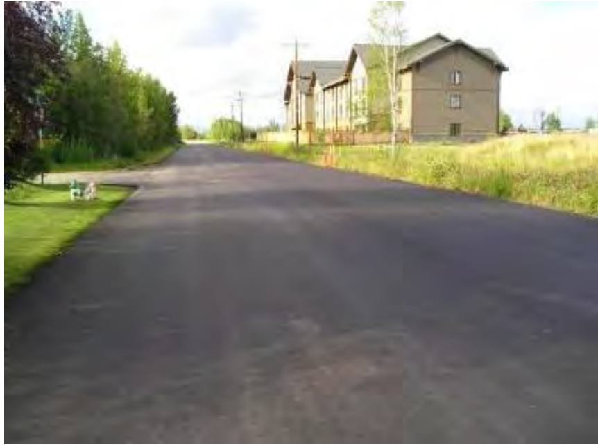
Figure 4-5. Finnell Dr, North Pole, just after thin HMA overlay, 2011
