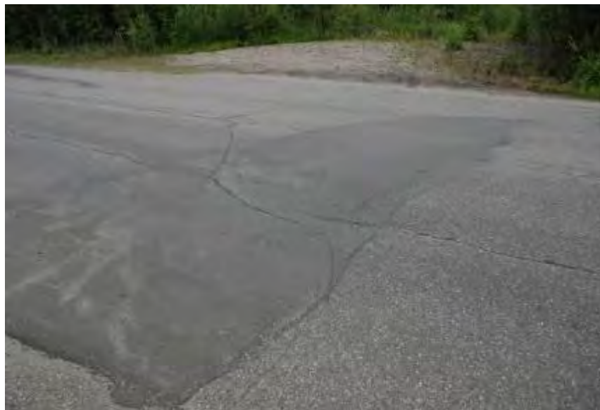
Figure 4-6. Cross Way, North Pole, just prior to thin HMA overlay, 2011
