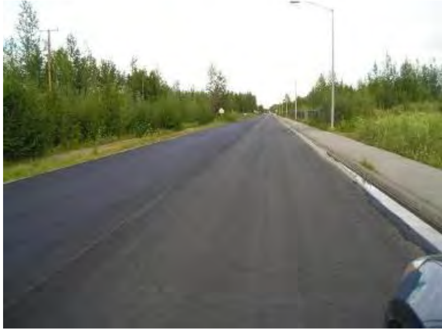
Figure 4-9. North Pole High School Boulevard, North Pole, just after thin HMA overlay, 2011
