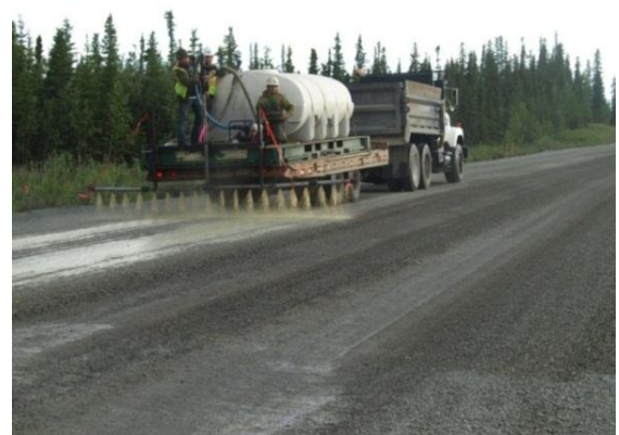
Figure 3 – Applying the palliatives with a 15' spray bar.
