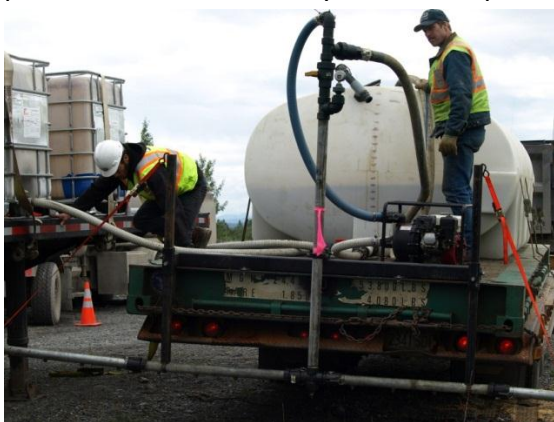
Figure 2 – Mixing palliative with water
