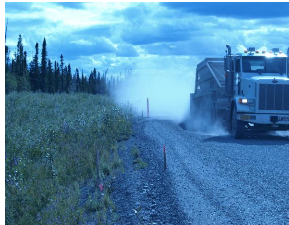
Figure 5 - Section 3B – 7/18/2011 – One Day after application of Soiltac
