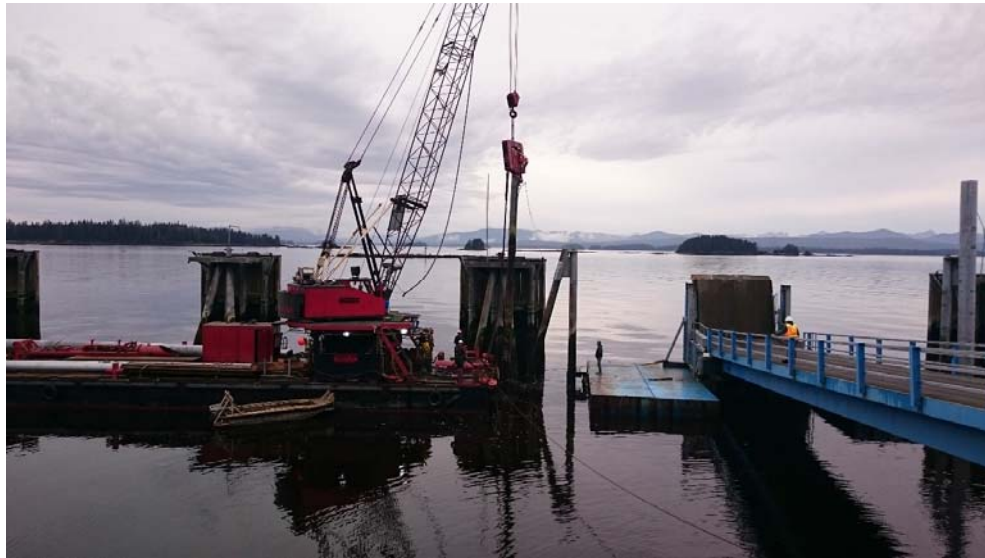
Vibratory pile driving at the Kake Ferry terminal (JASCO Applied Sciences, September 2015).
