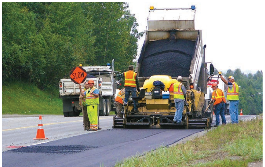
DOT Maintenance Crew Strip Paving DeBarr Road. Photo by Mark Parmelee, ADOT&PF
