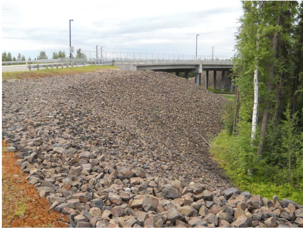
Air Conditioned Embankment, Thompson Drive, Fairbanks, photo by Jeff Currey, ADOT&PF
