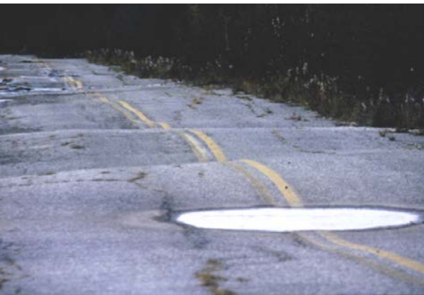
Effects of Permafrost on the Road Surface Photo by Mike Coffey ADOT&PF
