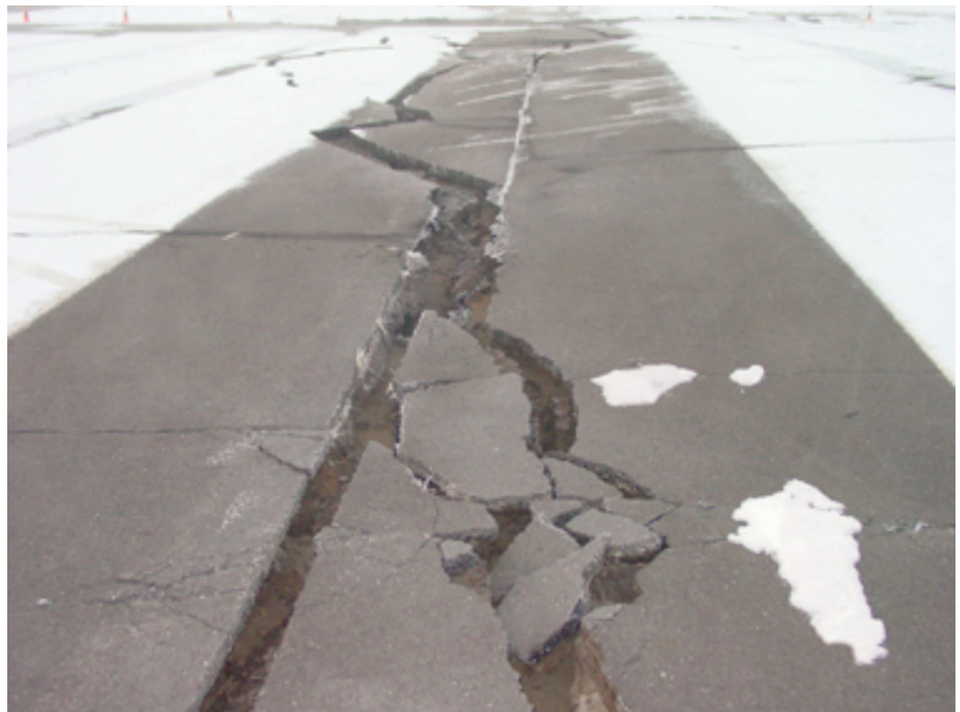
Earthquake Damage at the Northway Airport; photo courtesy of the Federal Highway Administration
