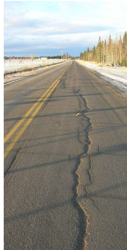
Cracking on the Funny River Road; photo by Jim Horn, ADOT&PF
