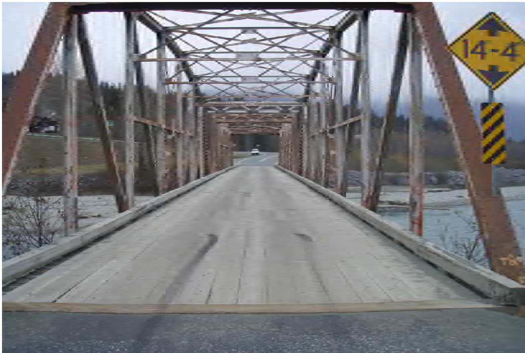
Figure 1a –Existing Steel Truss Klehini River Bridge. Looking east toward the Haines Hwy.
