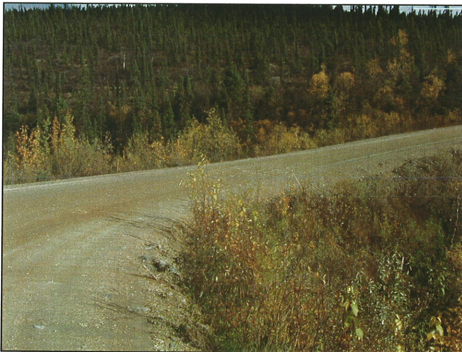
Photo 2. Typical road bed surface, MP 91 Taylor Highway (9/11/02).
