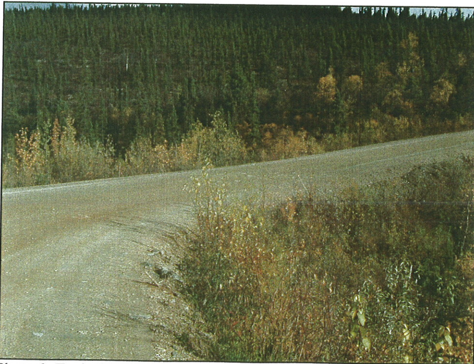
Photo 6. Typical road bed surface, MP 91 Taylor Highway (9/11/02).
