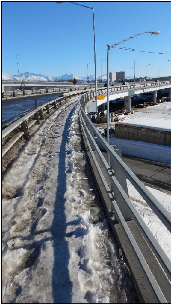
Figure 4: Sidewalk on C Street Bridge
